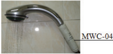
Fig. 11 Installation of MWC-04 as Magnetic Shower Adapter
